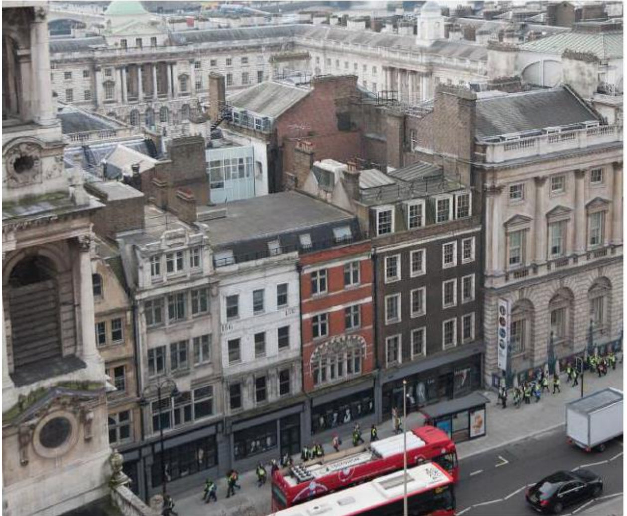
152-158 Strand front elevation from the roof of Bush House
